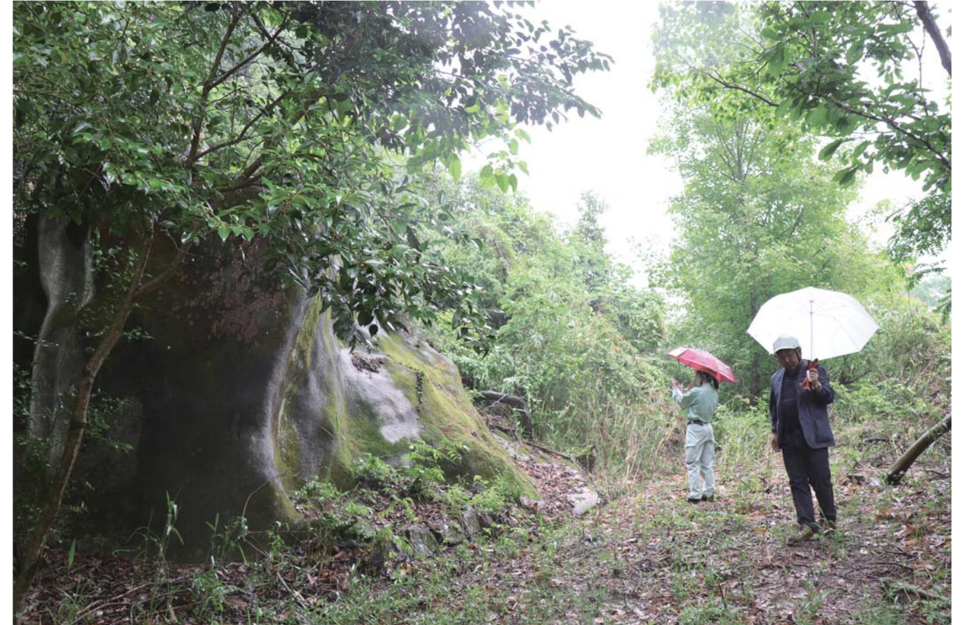
We patrol suspended and closed mines on a regular basis. If we find a new caved-in hole, it will be plugged or enclosed by fences to prevent people from falling. There are numerous aspects to check to see whether closed pits are solidly closed, whether drain channels are working well and whether water is springing from a closed mine.
